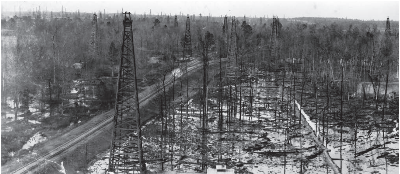
More than 75 derricks are shown drilling the field in Smackover, Arkansas, 1925. The large number of wells drilled too closely together caused damage to the natural resources above and below the surface. Arkansas Museum of Natural Resources (1985.016.001).
